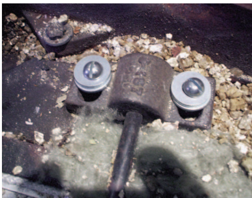
FIG. 5 USE LONGER FIXINGS
