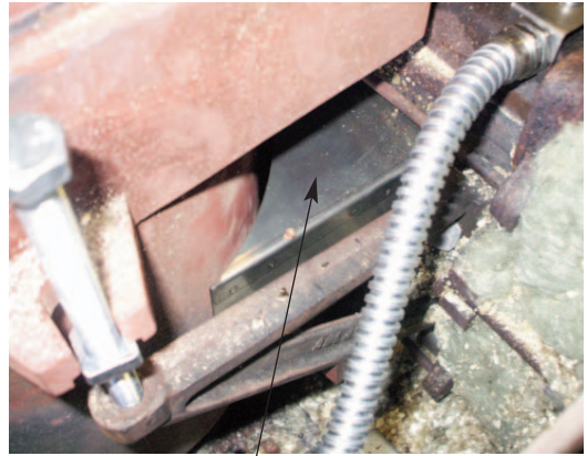
FIG. 4 FIT TUNNEL BETWEEN BARREL & OVEN
