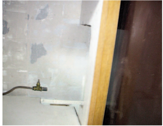
FIG. 2 CAP OFF OIL SUPPLY
