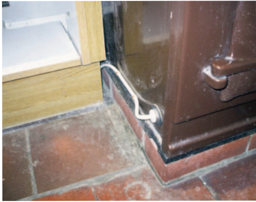
FIG. 5 ROUTE CABLE USE 'P' CLIP AND GROMMET
