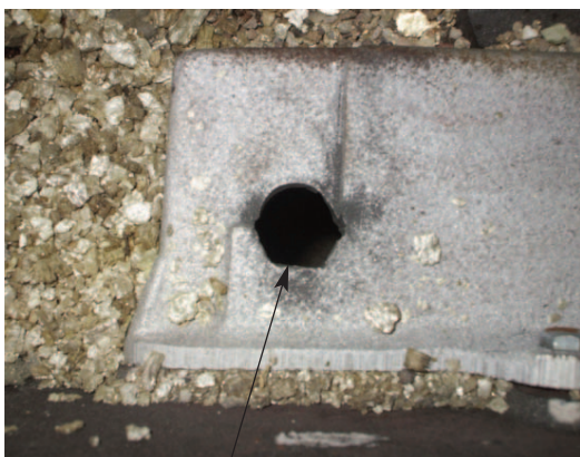
FIG. 3 MODIFY HOLE FOR FLEX CONDUIT FITTING
