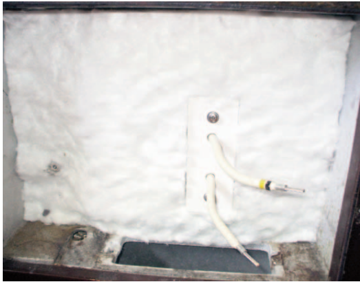
FIG. 2 FIT INSULATION BLANKET
