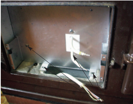
FIG. 3 FIXINGS FOR CONTROL BACK COVER
