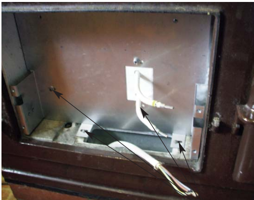
FIG. 3 FIXINGS FOR CONTROL BACK COVER
