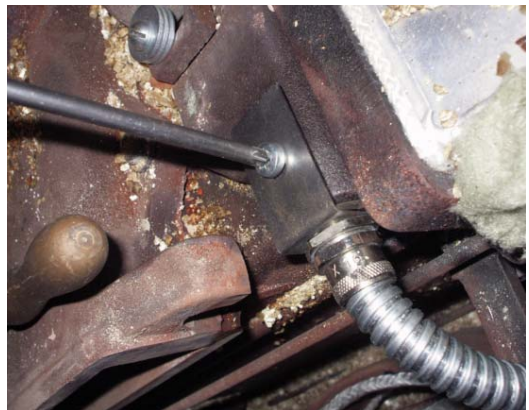
FIG. 4 FIT LOCATION BRACKET TO TOP OVEN
