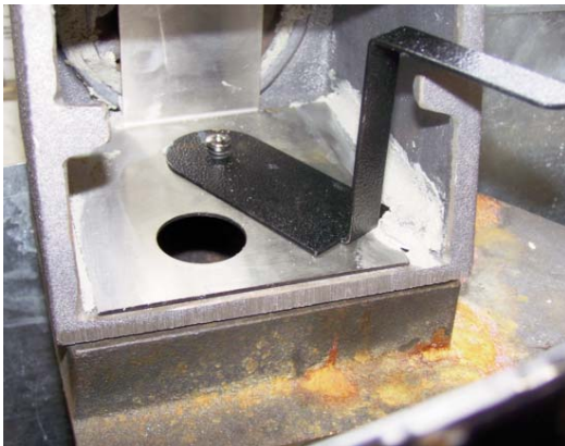
FIG. 5 POSITION AND FIRE CLAY IN PLACE
