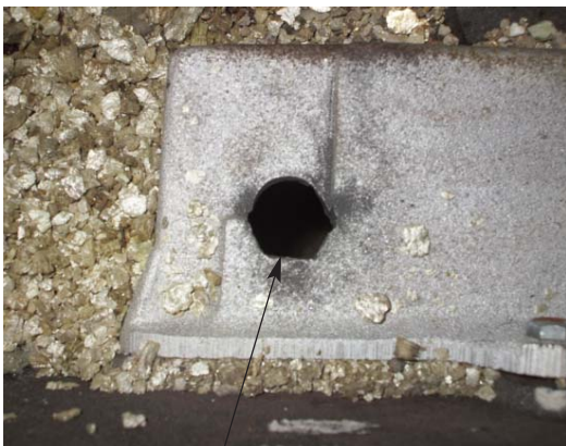
FIG. 3 MODIFY HOLE FOR FLEX CONDUIT FITTING
