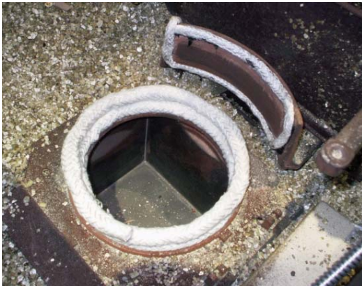
FIG. 3 FIT NEW ROPE SEAL
