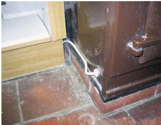
FIG. 5 ROUTE CABLE USE 'P' CLIP AND GROMMET
