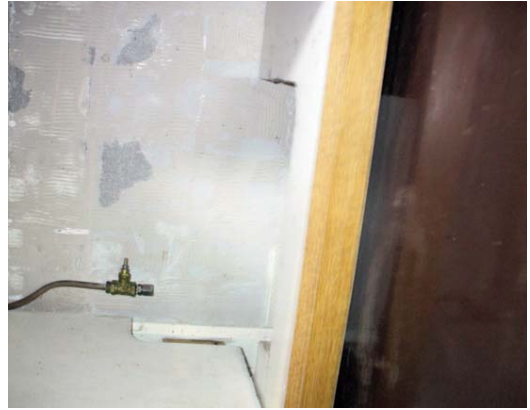
FIG. 2 CAP OFF OIL SUPPLY
