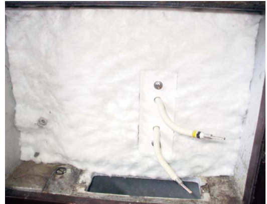
FIG. 2 FIT INSULATION BLANKET
