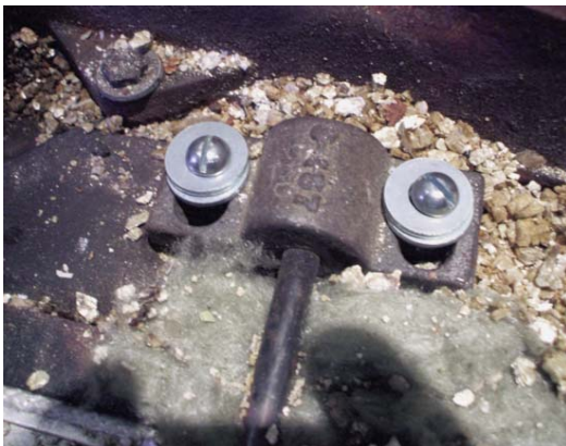
FIG. 5 USE LONGER FIXINGS
